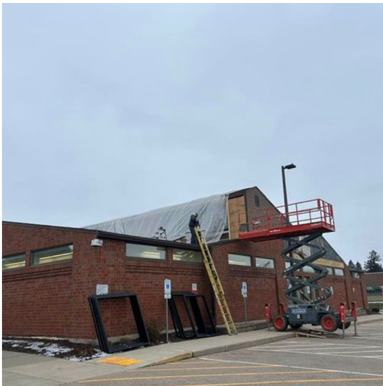
Clerestory window replacement for end of life windows is nearing completion.
