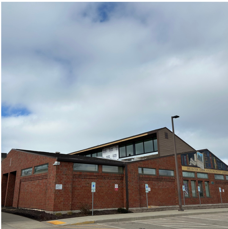
Clerestory window replacement completed. Roof installation scheduled to begin March 18.
